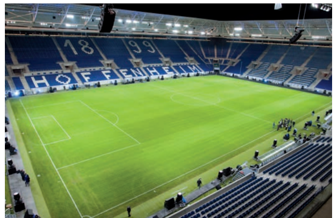
The roof structure of the football stadium belonging to TSG 1899 Hoffenheim mounted using GEDORE cordless torque wrenches.
